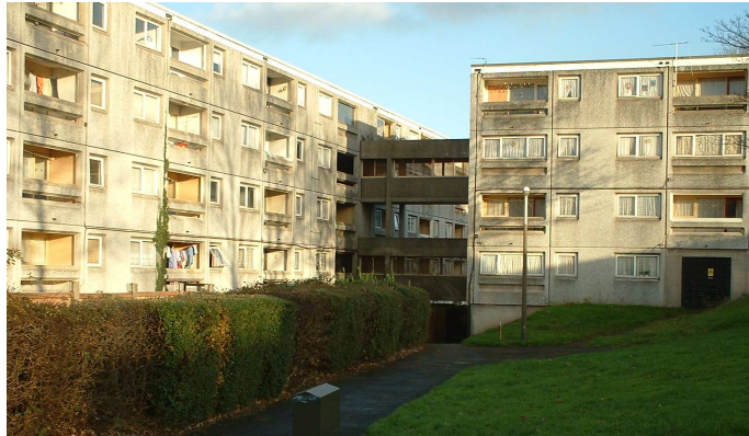
Photo 1 – Example of deck-access flats
